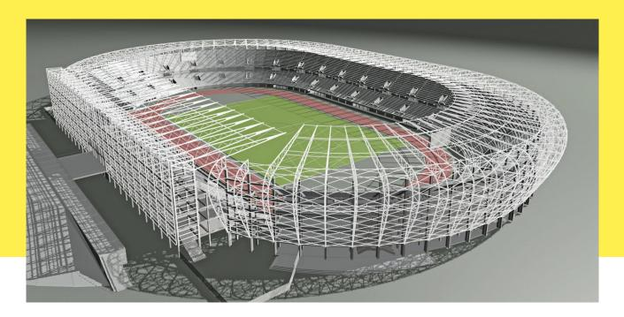
The erection of this steel structure was created within two steps. The first step was the erection of a pre-fabrication hall with a length of 170 m to finalize the steel girder for the assembling on-site and the assembling of these components and the roofing.
